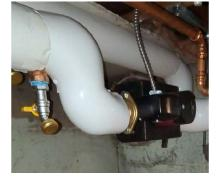
Villa Anginette Apartments worked with Rhode Island Energy to install over 400 linear feet of heating and domestic hot water pipe insulation.
