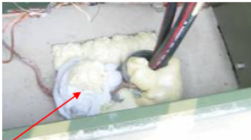
To seal spare conduit , install rag and fill with the expanding foam.
