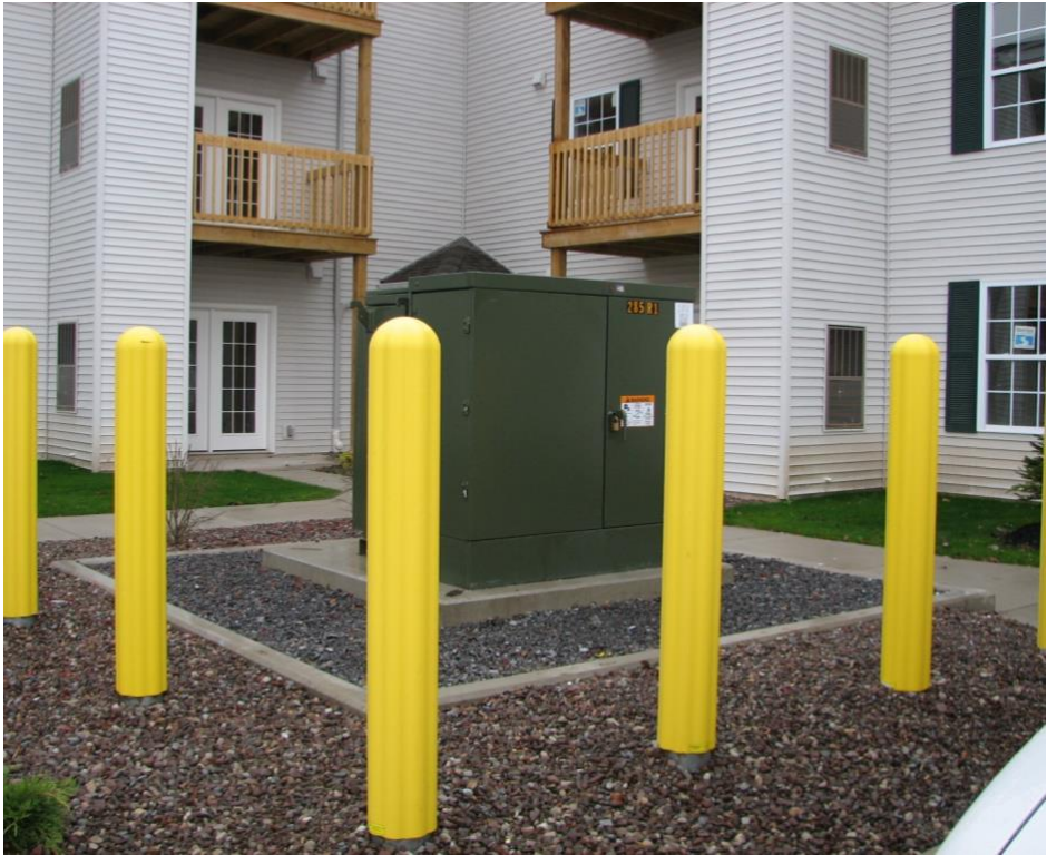
Picture of Ballard Installation
